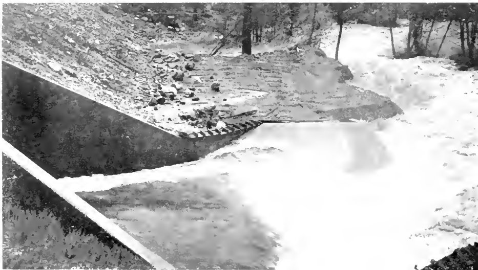
FIG. 35b. Close up of Salt Creek outlet, shooting at 22 feet per second
